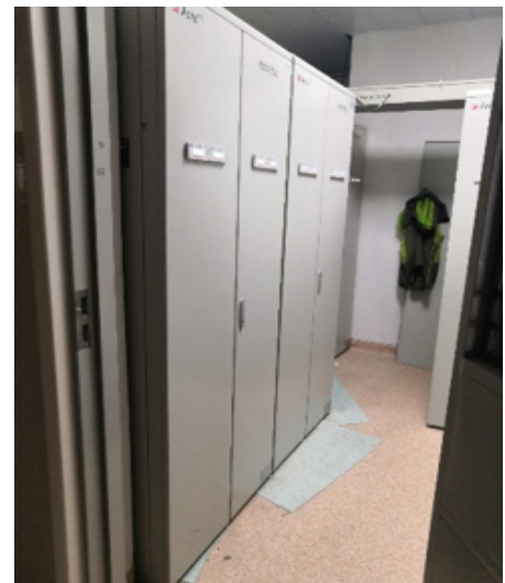
(2) Site Installation Picture
