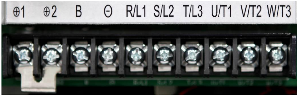
Diagram 4.1 Main loop connecting terminals
