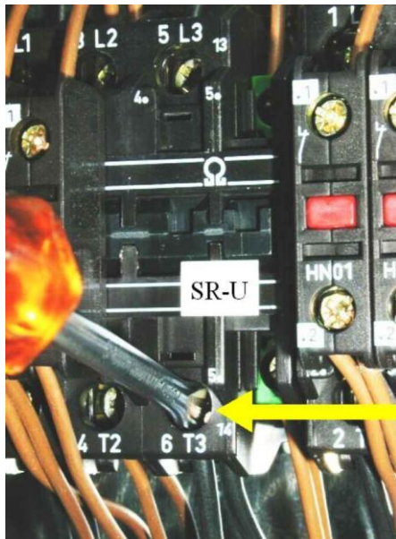
Retightening of Terminals
